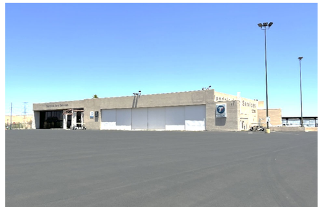
Glendale Aero Services (Terminal Apron)
